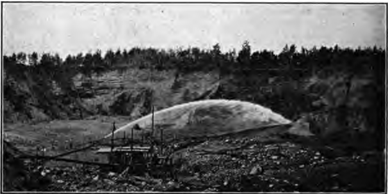
HYDRAULIC METHOD OF STRIPPING OVERBURDEN AT THE HILLCREST MINE, CUYUNA RANGE
